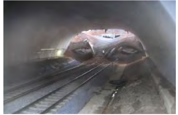
Gerrard's Cross cut-and-cover collapse, 2005 (View from inside the remaining tunnel)
