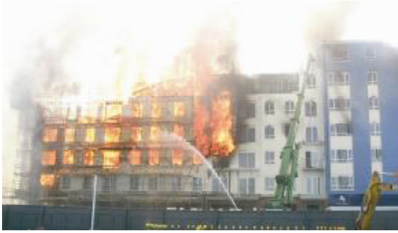
Colindale timber-framed fire, 2006 (courtesy London Fire Brigade)
