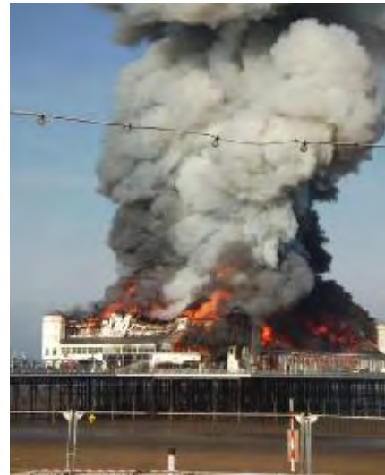
Weston-Super-Mare pier fire, 2008
